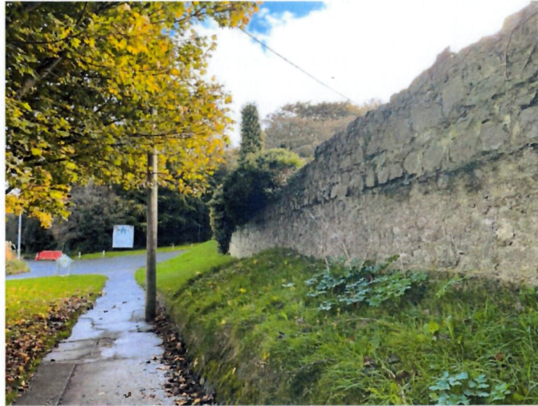
Close up view of the boundary wall within the Howth Castle ACA. A clear demarcation or rebuild can be seen along with ivy and other vegetation on wall as it curves south towards the entrance gate to the castle.
